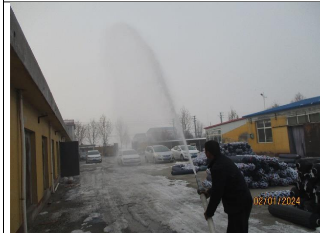
Fire hydrant testing
